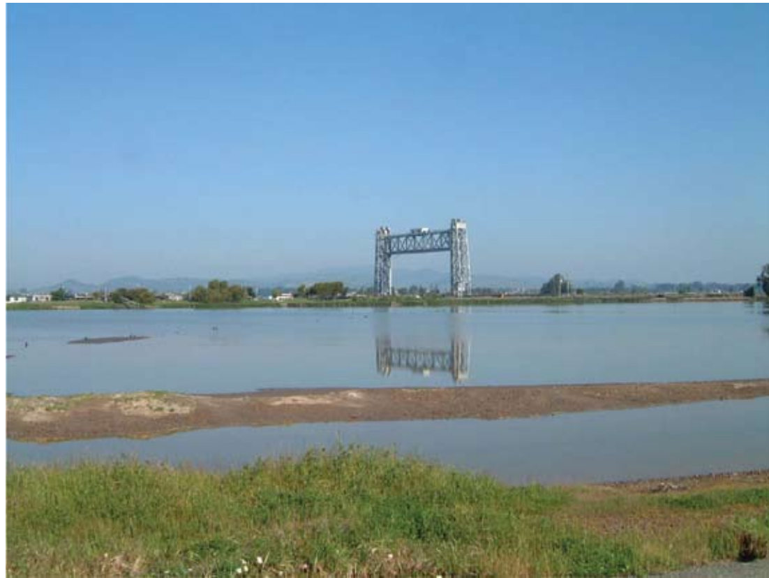
Photo 1. Wash Pond (W1), April 2005 (looking northwest).
