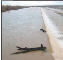
Raising the height of this outlet weir is one of a number of possible improvements to a 1930s-era settling basin where Cache Creek empties into the Yolo Bypass near the city of Woodland. The basin traps an estimated half of the mercury coming downstream in wet years.
