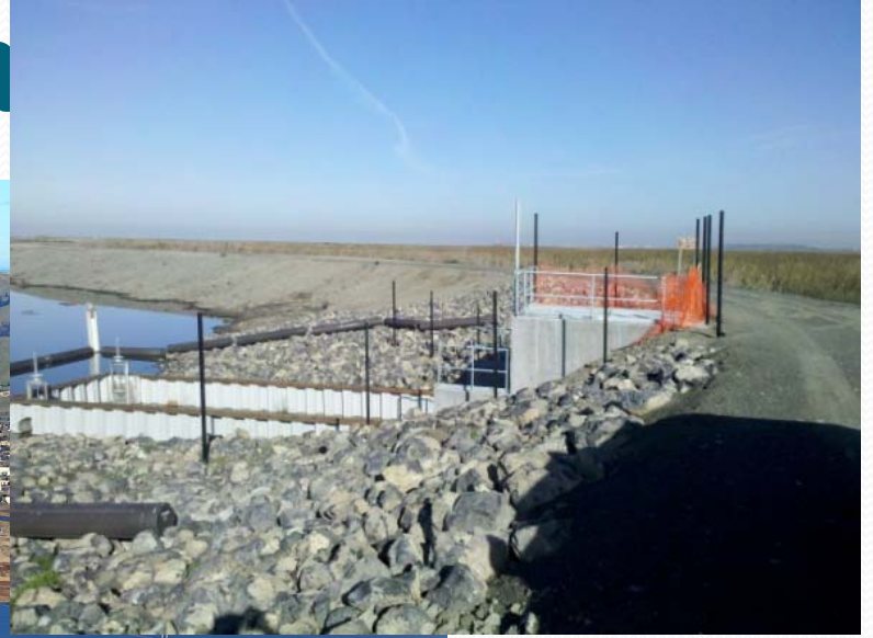
A16 outlet structure on inside of pond – weir box
