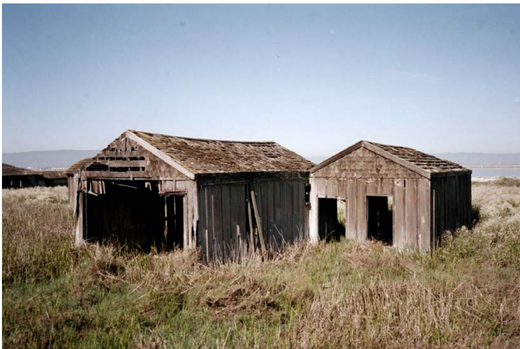
Figure 20. Drawbridge buildings (FWS 2002-05-09:01).
