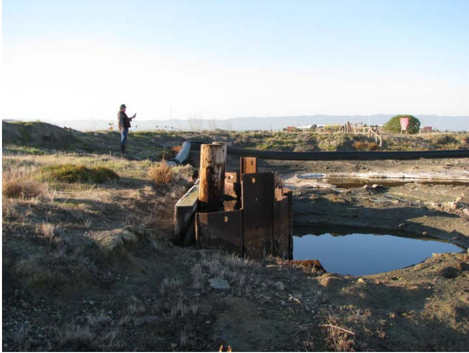
Figure 26. Water control structure and siphon/pipe extending beneath freeway to south (2007-12-01:152).
