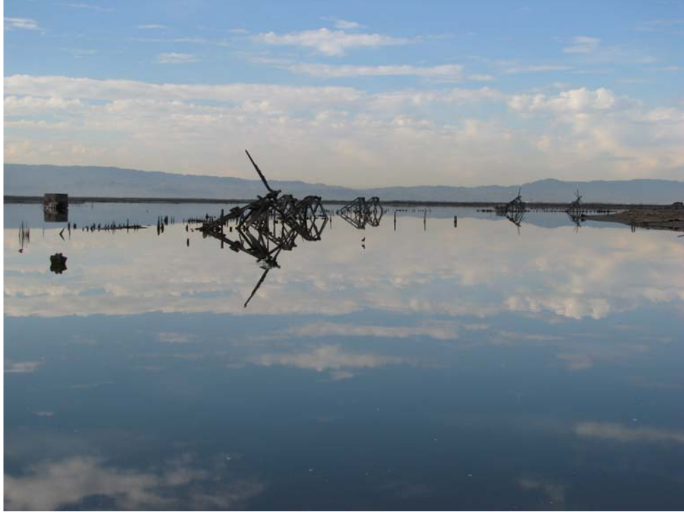
Figure 12. Archimedes screw pumps at Oliver Salt Works, view to W (2007-12-01:60). Note hunting blind in background.
