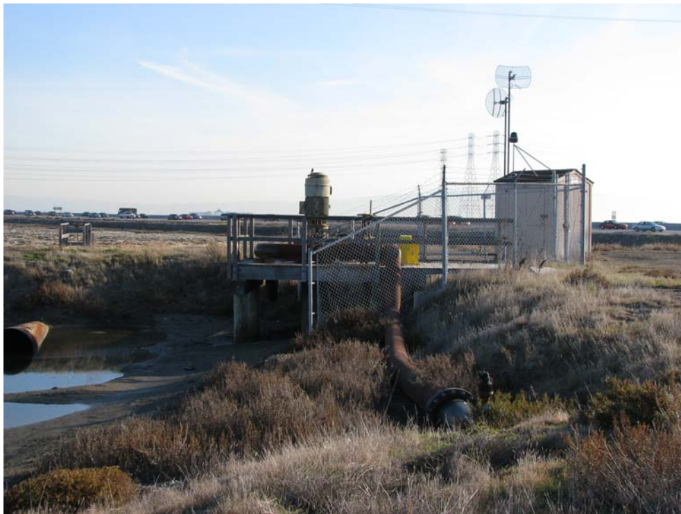
Figure 27. New pump station and pipes (2007-12-01:155).
