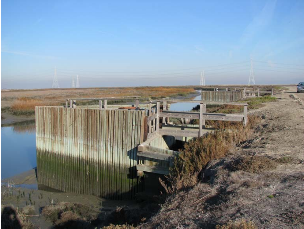
Figure 28. New water control structures on Ravenswood Slough side of levee (2007-12-01:163).
