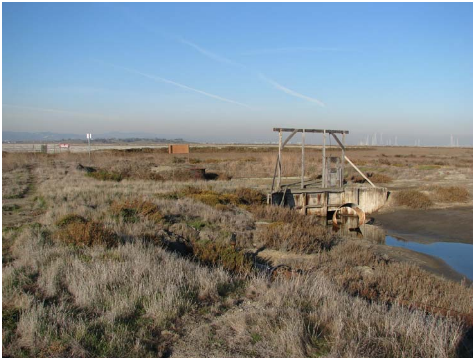
Figure 29. Abandoned water control structure, wooden headgate (2007-12-01:154).
