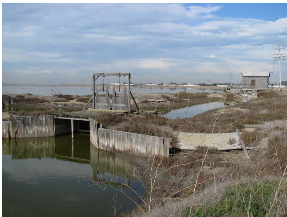
Figure 15. Water control structure, pump station, and powerline, all are non-contributing elements (2007-12-01:82).
