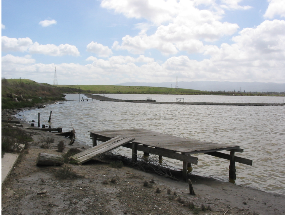
Figure 22. Temporary dock/landing in Alviso ponds, non-contributing elements (2007-03-04:108).
