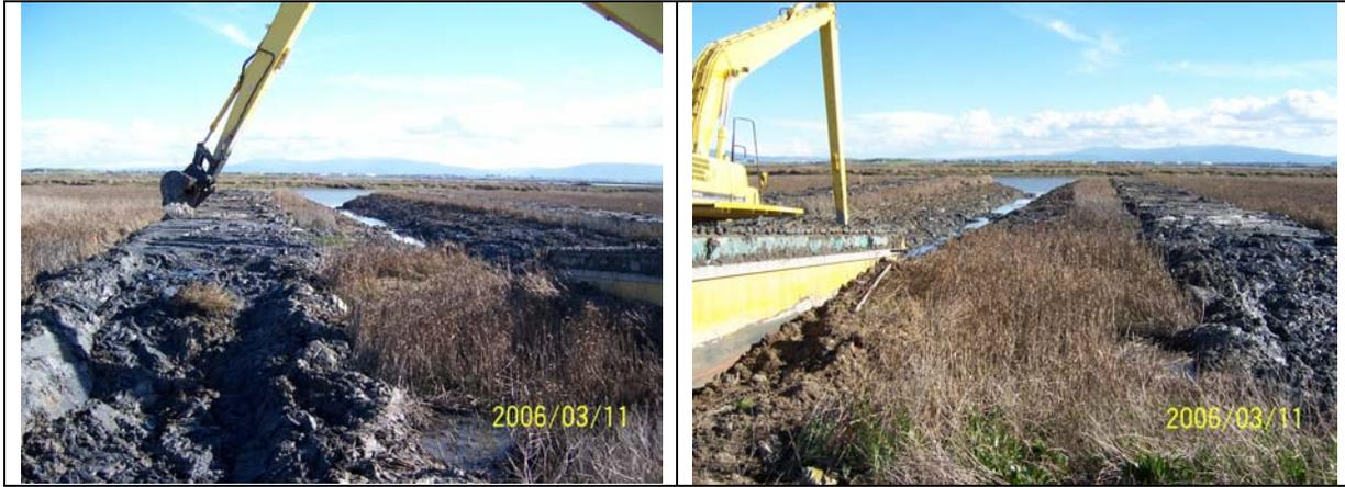
Pond A20 sidecast berm construction, looking towards Coyote Creek from old levee
