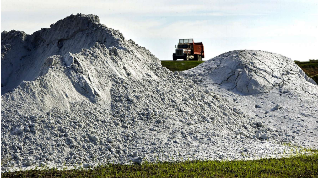
Lime waiting to be spread along a levee at the Sears Point Wetland Restoration, which began with fanfare in 2015 but could take 15 years or more. Michael Macor, The Chronicle
