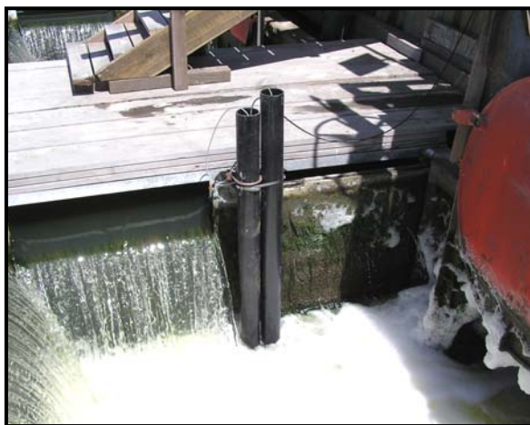
Figure 2-1: Datasonde within Weir Structure
