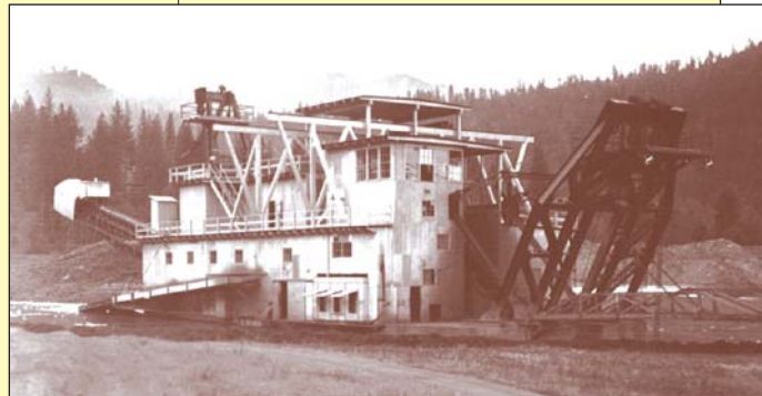
Gold mining dredge, Junction City district, Trinity River, 1935. Note the bucket line behind the gantry at the near end (right side) of the dredge, the stacker conveyor discharging coarse tailings at the far end, and the side sluice discharging fine tailings to the rear. The dredge separated the coarse material inside the housing, and fine material passed through sluices and over tables charged with mercury to capture the gold. Gold dredging occurred on more than a dozen Sacramento and San Joaquin river tributaries between 1898 and 1968, distributing mercury into the river system (see p.2).
