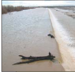
Raising the height of this outlet weir is one of a number of possible improvements to a 1930s-era settling basin where Cache Creek empties into the Yolo Bypass near the city of Woodland. The basin traps an estimated half of the mercury coming downstream in wet years.
