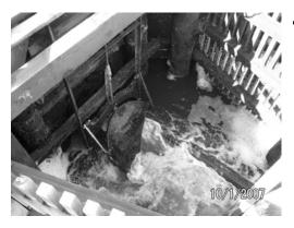
floating in pond crashed through flapgate breaking it and lodging in trash rack: uncontrolled release of water in pond
