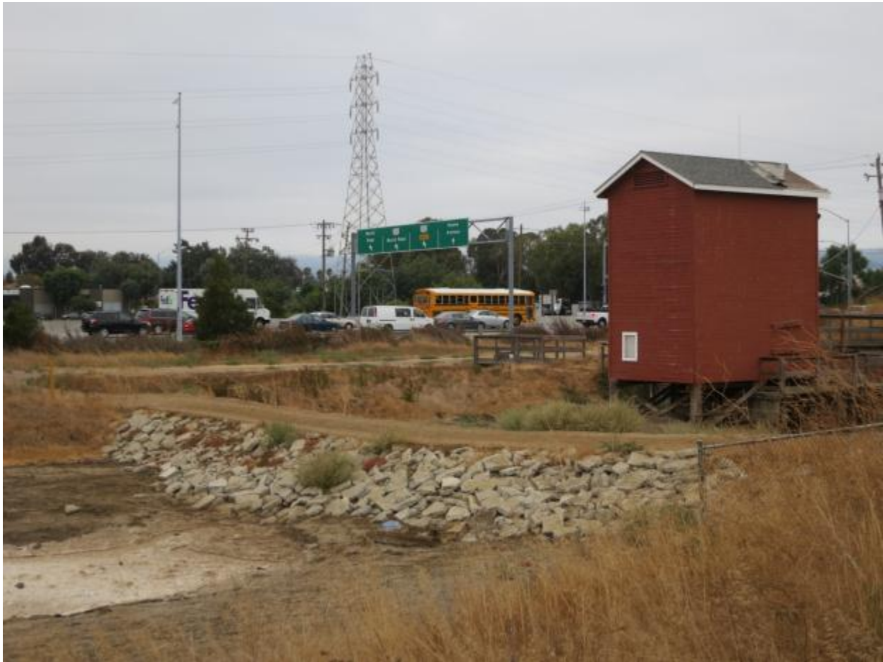
Figure 3.16-4. View of pumphouse, facing northwest from Bedwell Bayfront Park.
