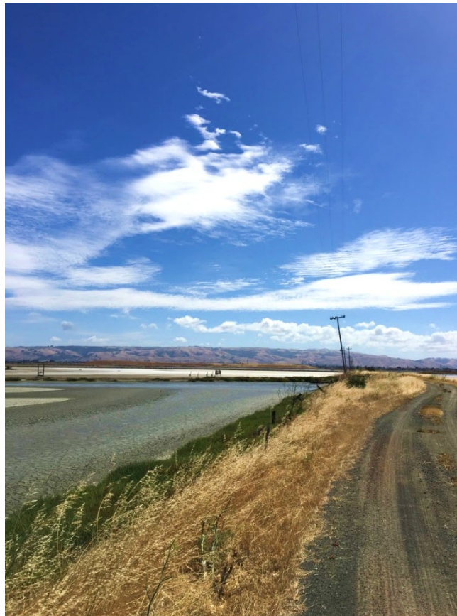
Figure 3.16-3. View from Levee Separating Ponds E5C and CP3C, Facing East
