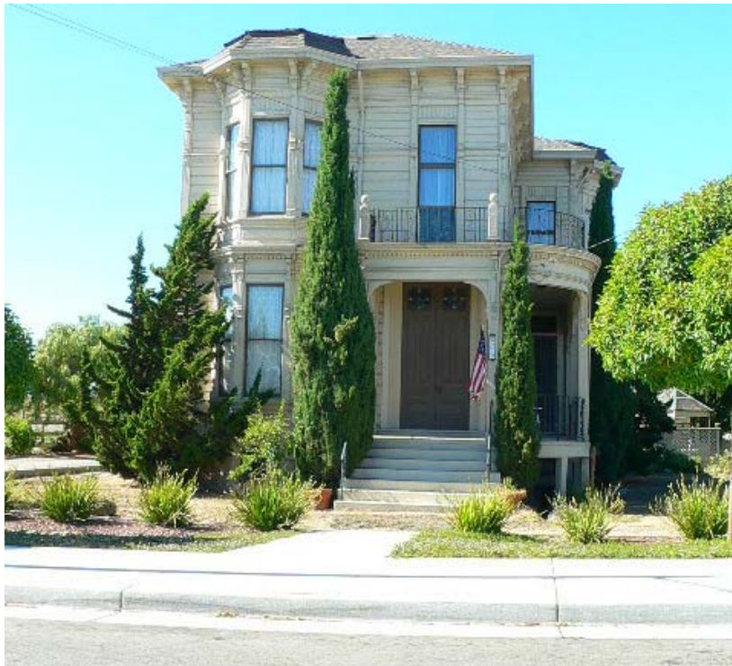
Figure 3.8-6 Tilden-Laine residence, Alviso, 2006
