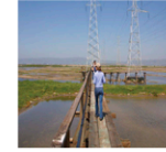
access to infrastructure
