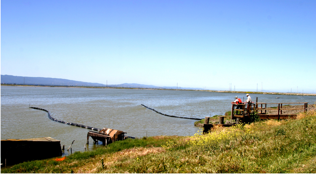
Figure 3-2: Baffles at Pond A3W discharge
