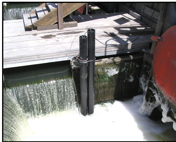
Figure 2-1: Datasonde within Weir Structure
