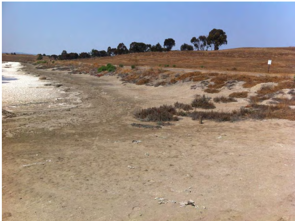
Figure 9v. Ravenswood Pond Levee Between R5 and R4 at the Southeast Corner of Bedwell-Bayfront Park Looking North (Salt Pond Jurisdiction area)
