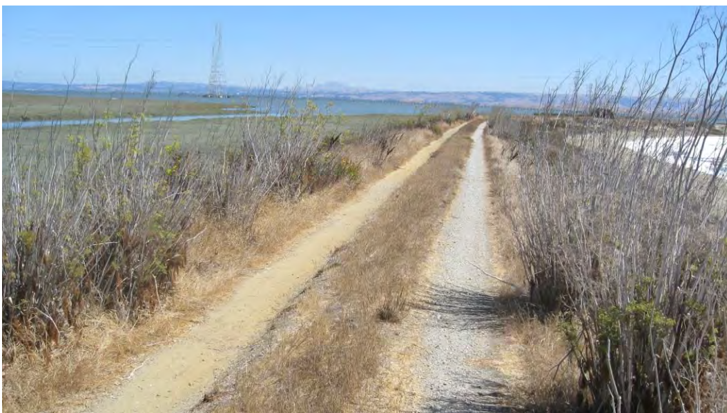
Figure 9t. Levee Between Westpoint Slough and Pond R4 (100-foot Shoreline Band Jurisdiction area)
