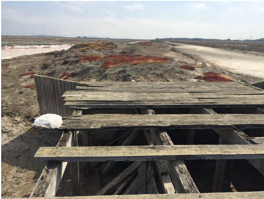
Figure 9y. View of norther levee of the All American Canal between Ponds R3 and R4 looking to the east with existing water control structure to be removed in the foreground. Location is near proposed R3/R4 viewing platform location (Salt Pond Jurisdiction).
