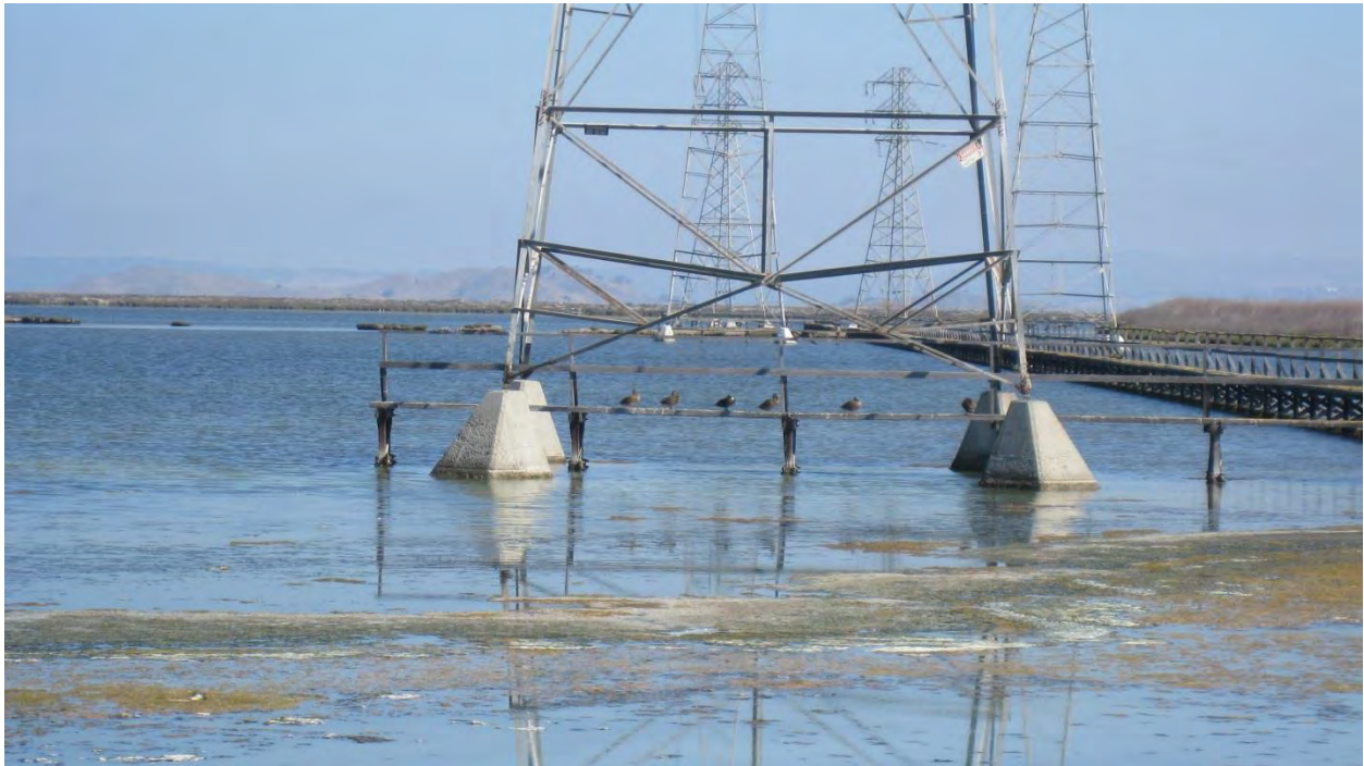
Figure 9o. Existing PG&E infrastructure (boardwalks and towers) in Pond A2W (Salt Pond Jurisdiction).
