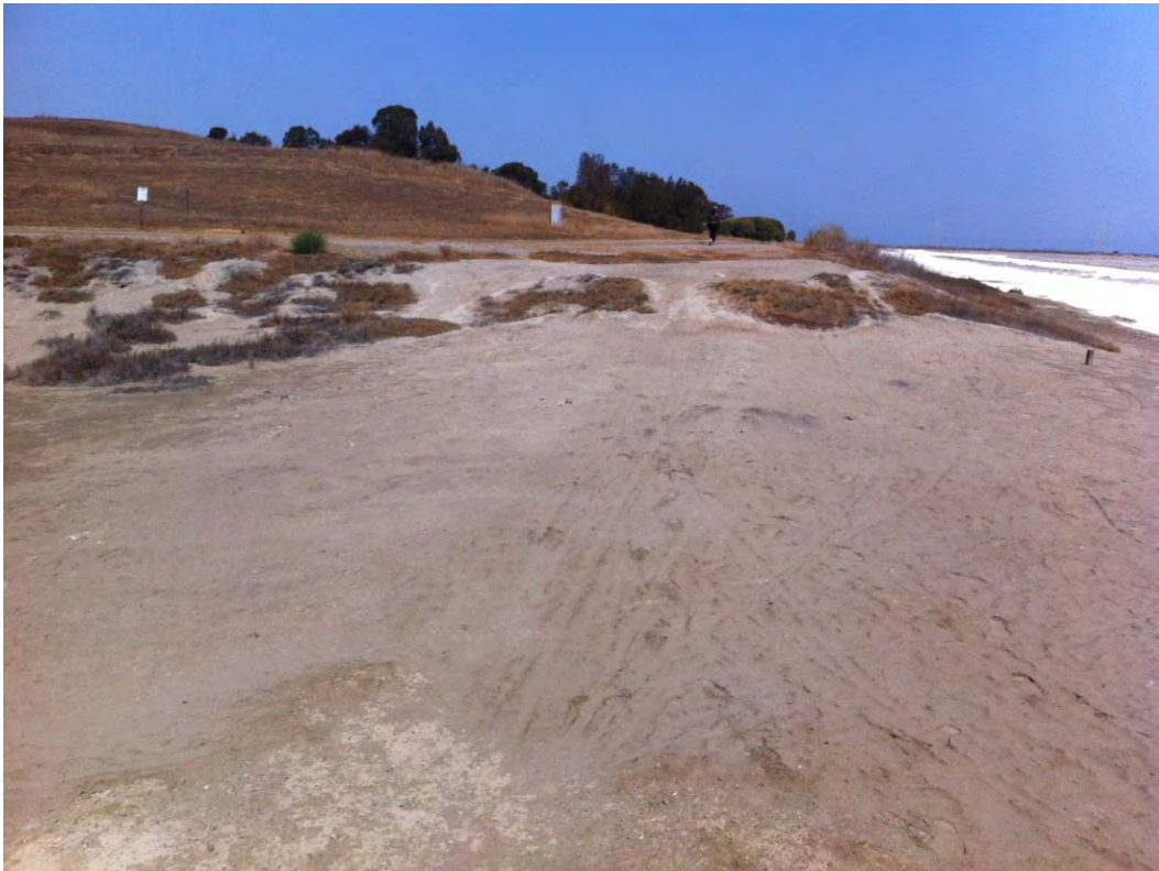
Figure 9s. Ravenswood Pond Levee Between R5 and R4 at the Southeast Corner of Bedwell-Bayfront Park Looking North (Salt Pond Jurisdiction area)
