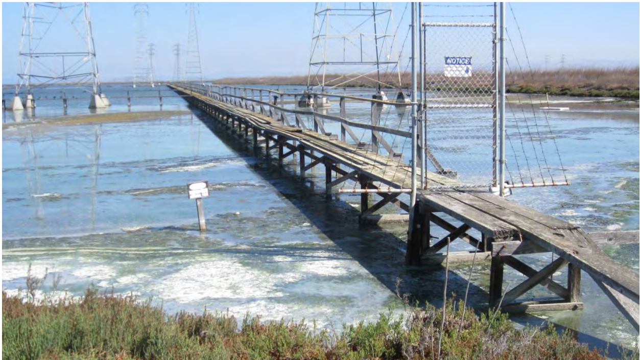
Figure 9p. Existing PG&E infrastructure (boardwalks and towers) in Pond A2W (Salt Pond Jurisdiction).
