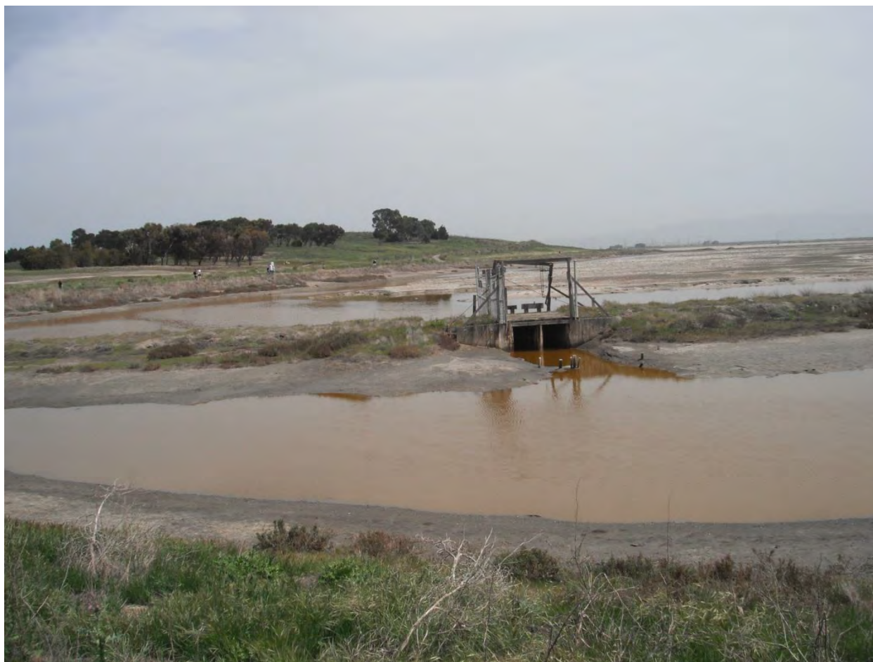
Figure 9z. Existing water control structure between ponds S5 and R5 to be removed (Salt Ponds Jurisdiction)
