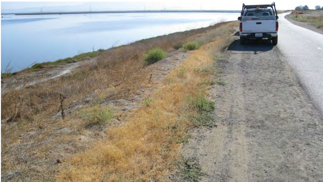
Figure 9j. Mountain View Pond A1 Shoreline as Viewed from the Bay Trail (Salt Pond Jurisdictional area)
