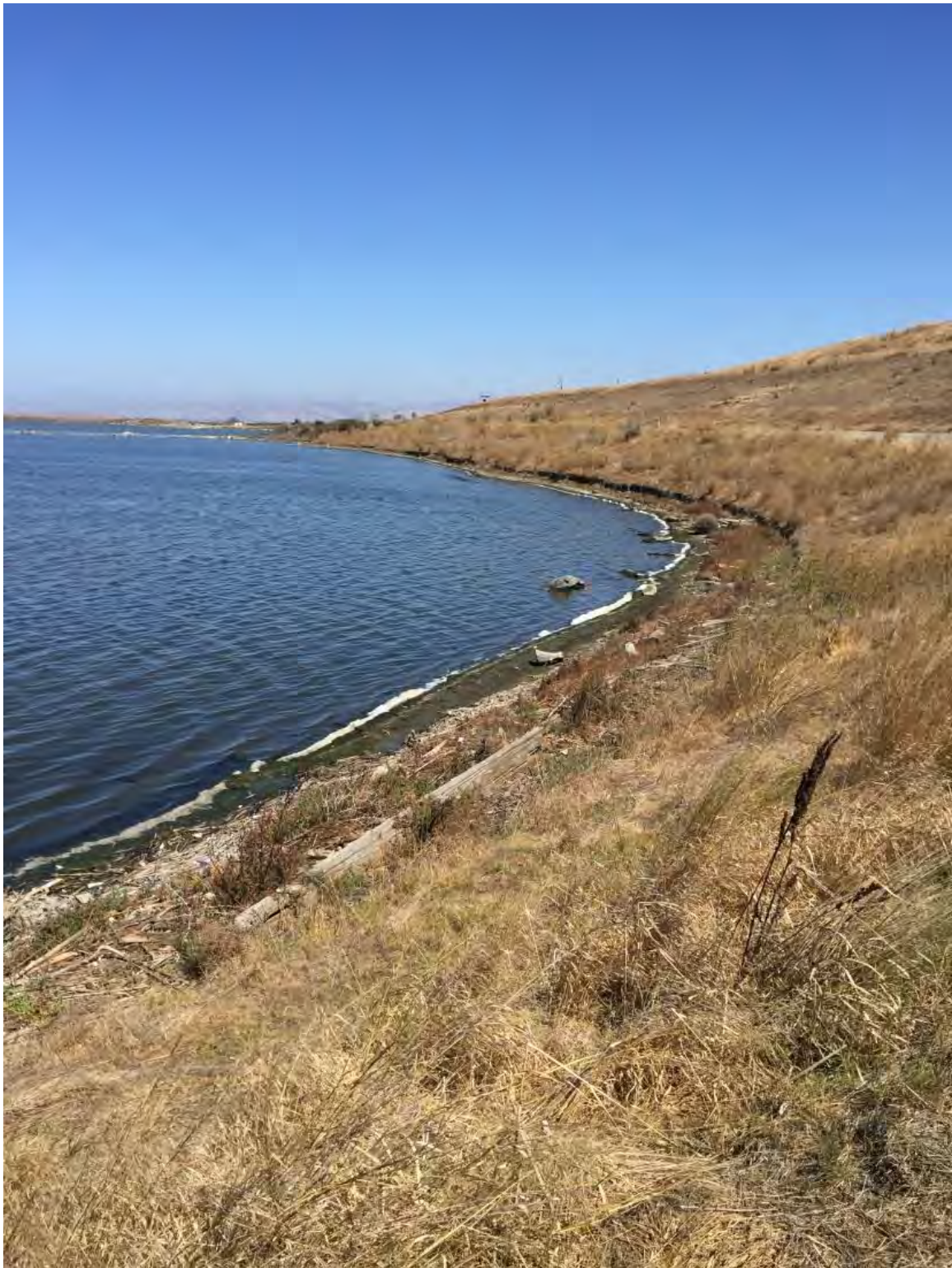
Figure 9g. Pond A8 Shoreline at Southeast Corner Where Habitat Transition Zone Would be Installed (Salt Pond Jurisdiction area)
