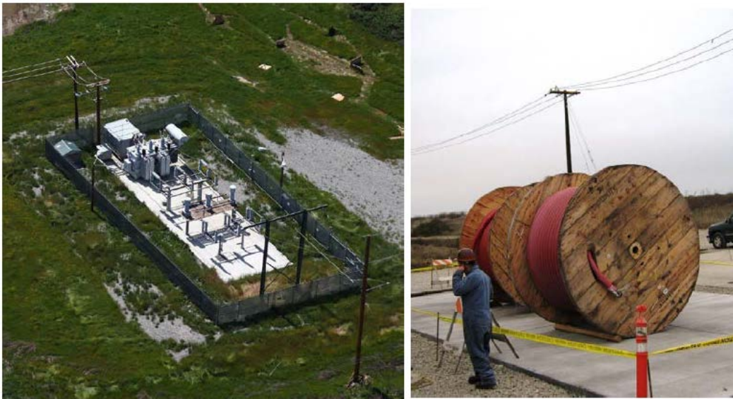
Figure 4.7. Electrical Substation and Submarine Power Cable used at Hamilton Wetlands Restoration Project
