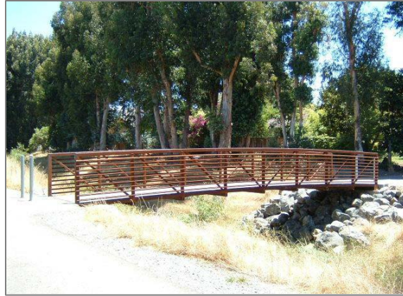
Figure 4.22 Representative Light-duty Bridge with Abutment Armoring
