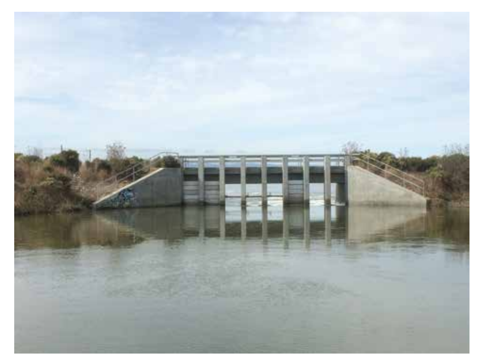
Flow-control structure at Pond A8. The opening of each 1.5-m-wide gate was phased to gradually increase tidal flows to the Pond A8 complex.
