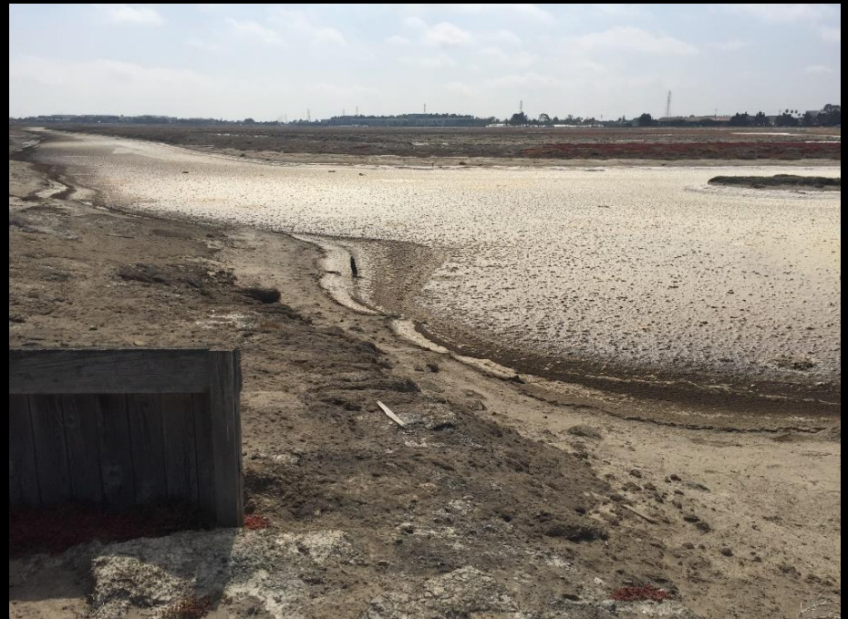
Soon-to-be restored marsh at Ravenswood Pond R4
