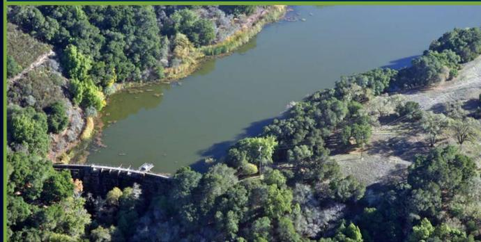
**SEARSVILLE DAM** Completed in 1892 and located within the Jasper Ridge Biological Preserve, Stanford University's 65-foot tall Searsville Dam has lost more than 90% of its original water storage capacity as roughly 1.5 million cubic yards of sediment have filled in the reservoir. The dam provides no potable water, no flood control, no hydropower, and only a small amount of water for irrigation.
