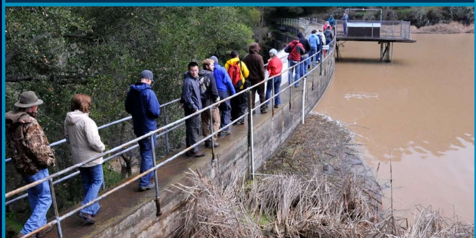
**SEDIMENT TRAP** For more than a century now, the dam and reservoir have blocked sediment and nutrients. The dam also traps woody debris and spawning gravel, which degrades creek habitat for a variety of native animals.
