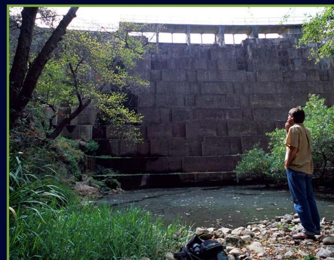
**DAMS DON'T WORK FOREVER** Stanford's own National Performance of Dams Program states that the "average age for a dam is 40 years." Searsville Dam is almost 120 years old. Large cracks on the dam were first observed in the 1930s. Its current structural condition is unknown, as it's been more than four decades since the California Division of Safety of Dams thoroughly inspected the foundation.
